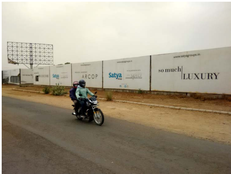
FENCING AROUND THE PROJECT SITE
