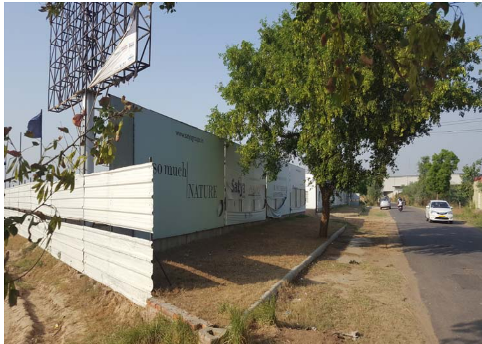
FENCING AROUND THE PROJECT SITE
