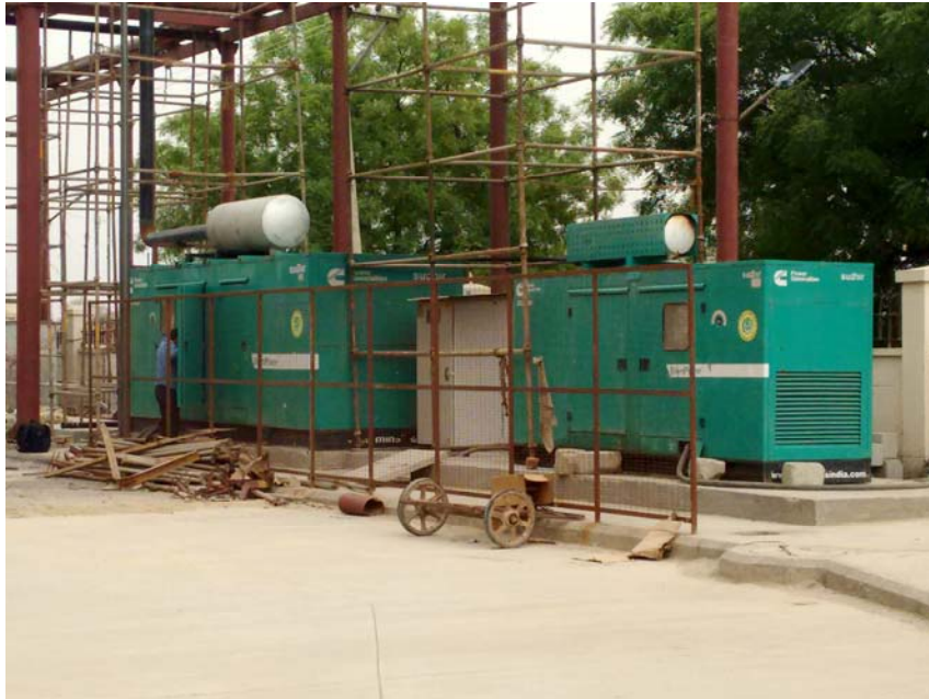
DG SETS UNDER INSTALLATION
