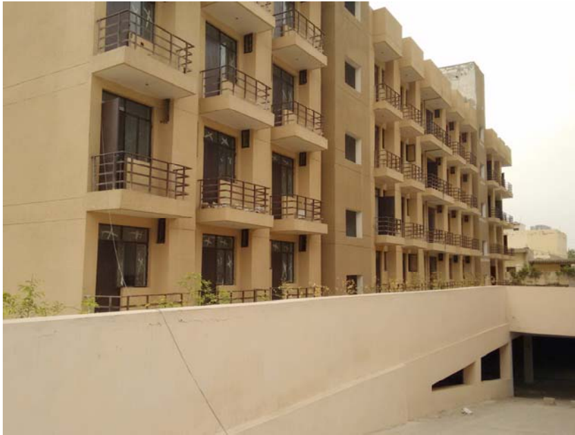
EWS FLATS AT CONSTRUCTION SITE
