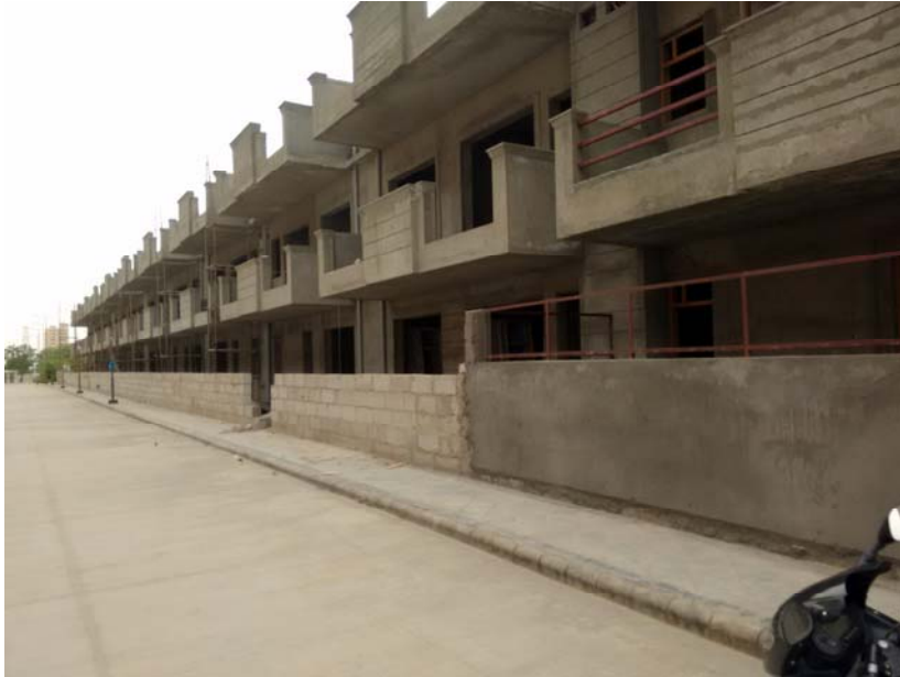
VILLAS UNDER CONSTRUCTION
